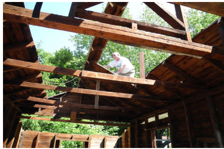
Tom Dutcher carefully prepares to take down the garage at the James St. Project where our mission team worked in WI in June. His leadership was a wonderful asset to the team.
