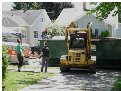
Emma Binkley, Karli Michaels bring debris from the basement to the dumpster. Dan Crowl assists in packing it.
