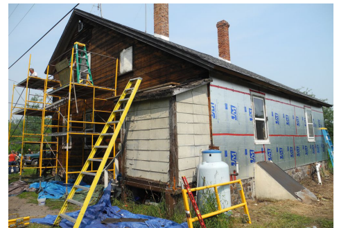
Team from Covenant Lutheran works to cover Baltic Project in R-board during their mission week in Keweenaw.
